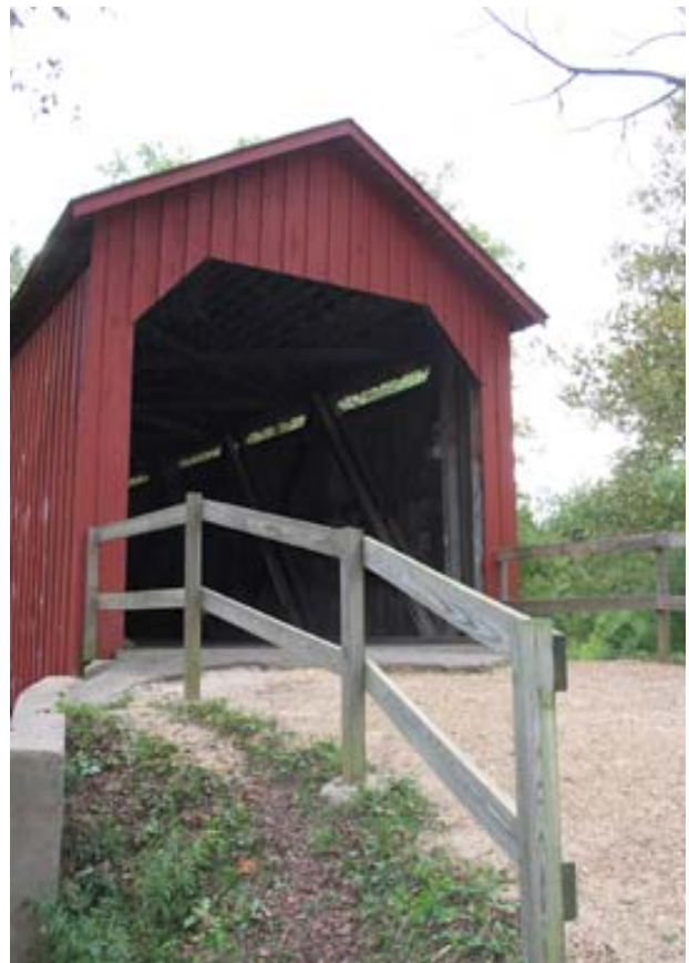
Another Picture from the Sandy Creek Covered Bridge
